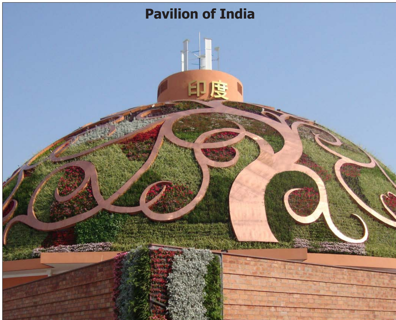
This rooftop photo shows grass and flowers on top of a membrane, which covers the bamboo dome below.
